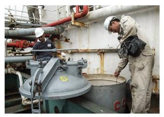
Figure 5: Testing the atmosphere of the enclosed space
